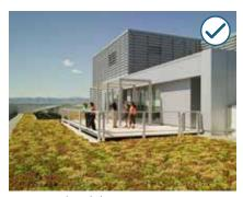
Design building projects to reduce stormwater runoff by including a greenroof.
