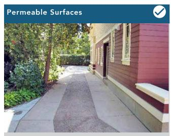
Permeable surfaces include paving systems that allow rainwater to percolate into the ground underneath. They can significantly reduce runoff from parking areas, drive aisles, pedestrian paths and plazas.
