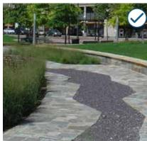
Incorporate Low Impact Development (LID) principles, such as stormwater planters and permeable pavement, to mitigate stormwater impacts.
