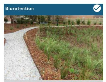
Bioretention systems manage and treat stormwater runoff in a shallow depression filled with a soil bed and planting materials to filter runoff. They help provide greater site utilization and attractive landscape areas while protecting water quality.
