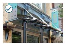
Use an architectural element(s) to highlight an entrance, and to provide weather protection, where feasible.
